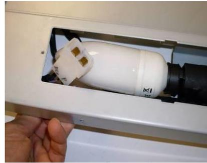
Figure 9: Passing cable through
