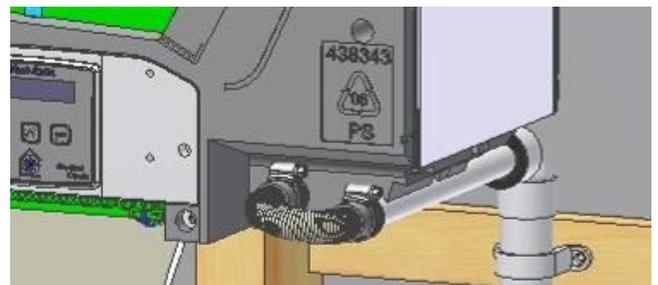
**N.B. Always insulate condensate pipe if installing in a cold void**
