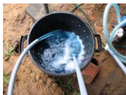
Fig 23 Purging the Slinkies of Air
