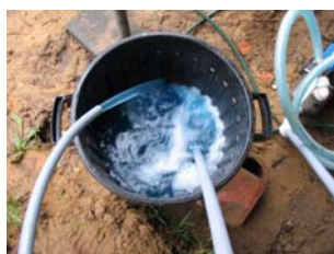
Fig 26 Purging the Slinky of Air
