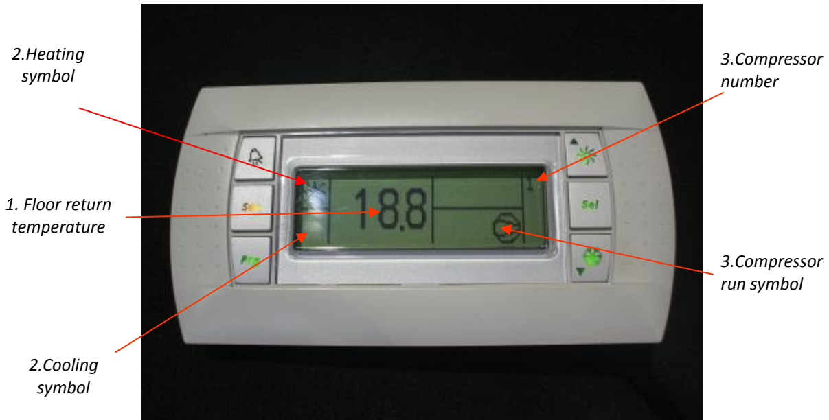
Fig 30 Heat Pump Display
